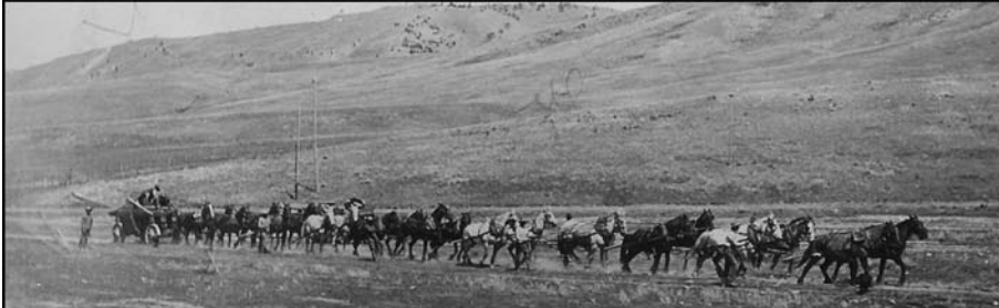
Upper Left: One of the rotor / turbines for the Madison River Power Plant. Upper Right: Rotor on the scow. Middle Right: Madison River Dam & flues. Above Right: Completed power plant Above: 25 horses and five men move the rotor up the Madison valley. Right: The interior of the power plant. Left: Street lamp on the corner of Cedar and Main St. Three Forks, c. 1917
